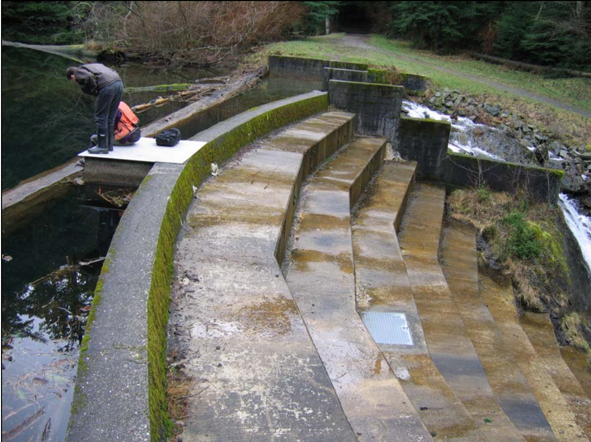
Mountain Lake Dam, February 2005
